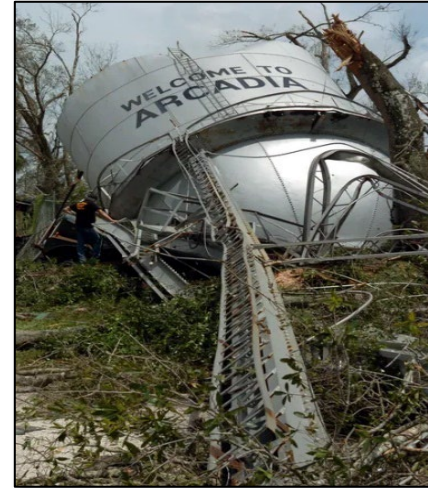
Figure 13: Fallen Water Tower in Arcadia from Hurricane Charley in August 2004 (Mott, 2014)
